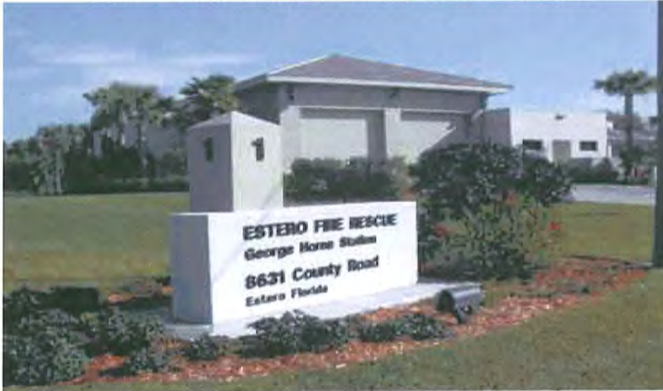
Figure 18: Estero Fire Rescue Station 1 – 8631 County Road
