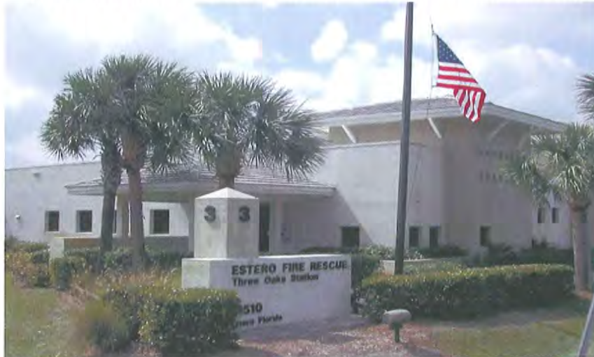
Figure 25: Esterio Fire Rescue Station 3 – 21510 Three Oaks Parkway
