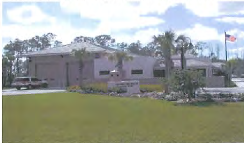
Figure 28: Estero Fire Rescue Station 4 – 21300 Firehouse Lane
