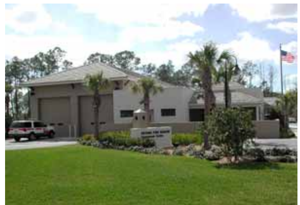
Station 4 – 21300 Firehouse Lane
