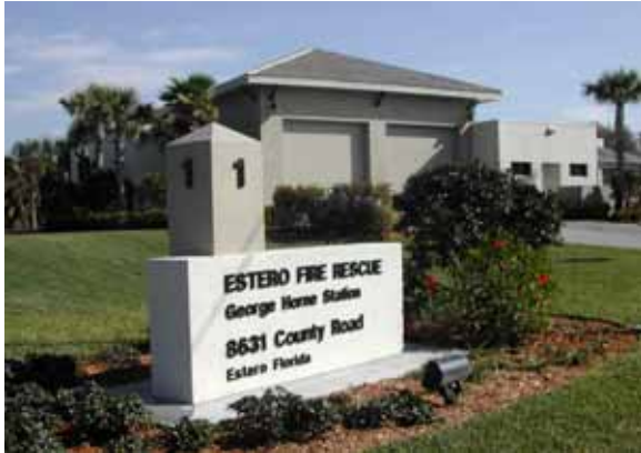
Station 1 – 8631 County Road
